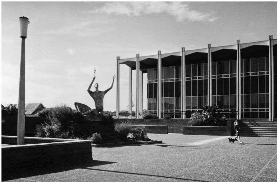
Figure 11: A view dated to 1967 of the Administration building which defined the eastern edge of an urban landscape of plazas and flower beds. Source: BL, 0001186
