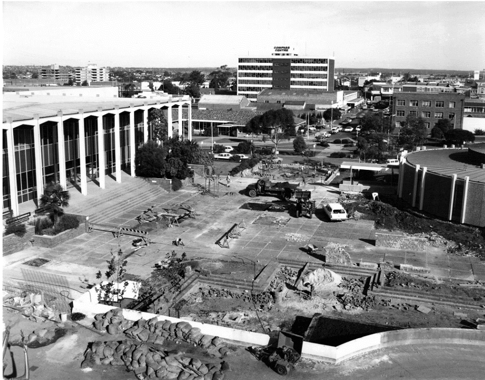
Figure 10: A view dated to the early 1960s showing the relationship between Bankstown's civic precinct (under construction) and the retail and commercial office uses on the development site. Source: BL, 27320
